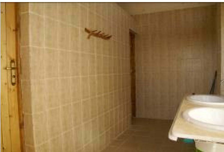
Beginning Oct 2008 – bathroom
