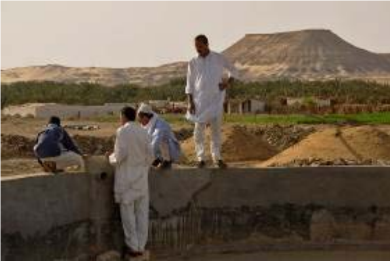
April 2008 – making the water pit
