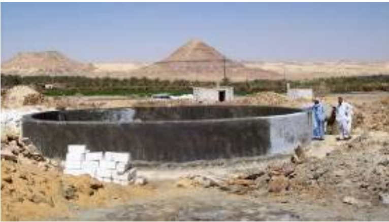
April 2008 – water pit almost finished
